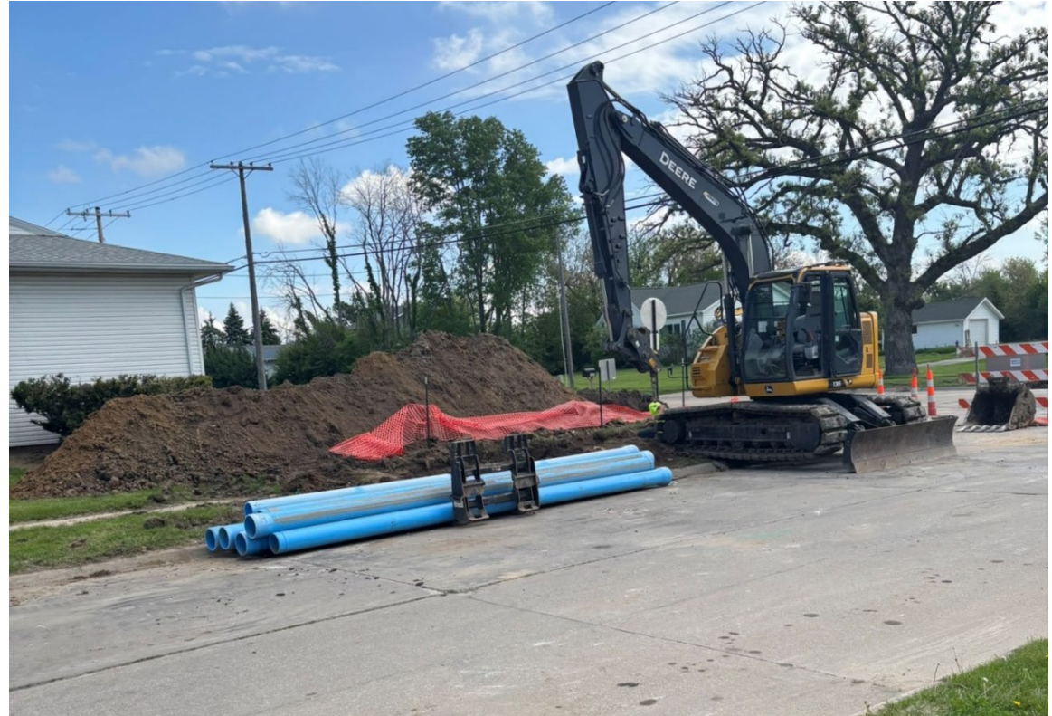
Photo: 5/13/2025, water main installation on Clymer Rd. in Hiawatha
