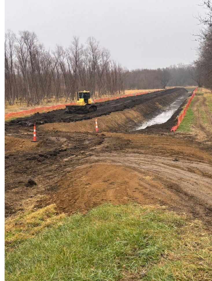
Photo: 11/24/2025, levee earthwork to install new force main
